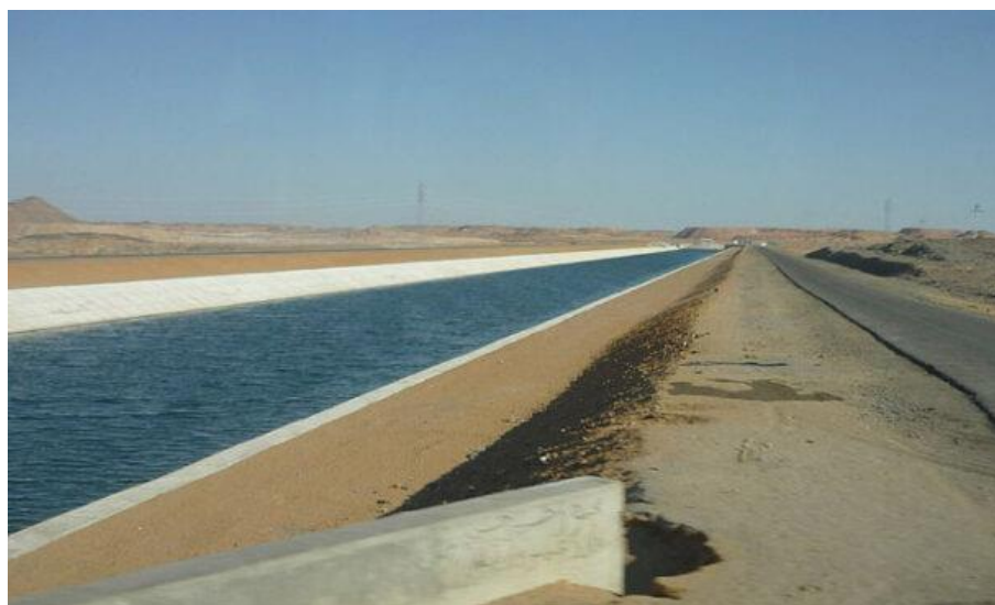
View of the canal delivering water from the Nile to the Toshka Lakes (photograph: Rémi)
