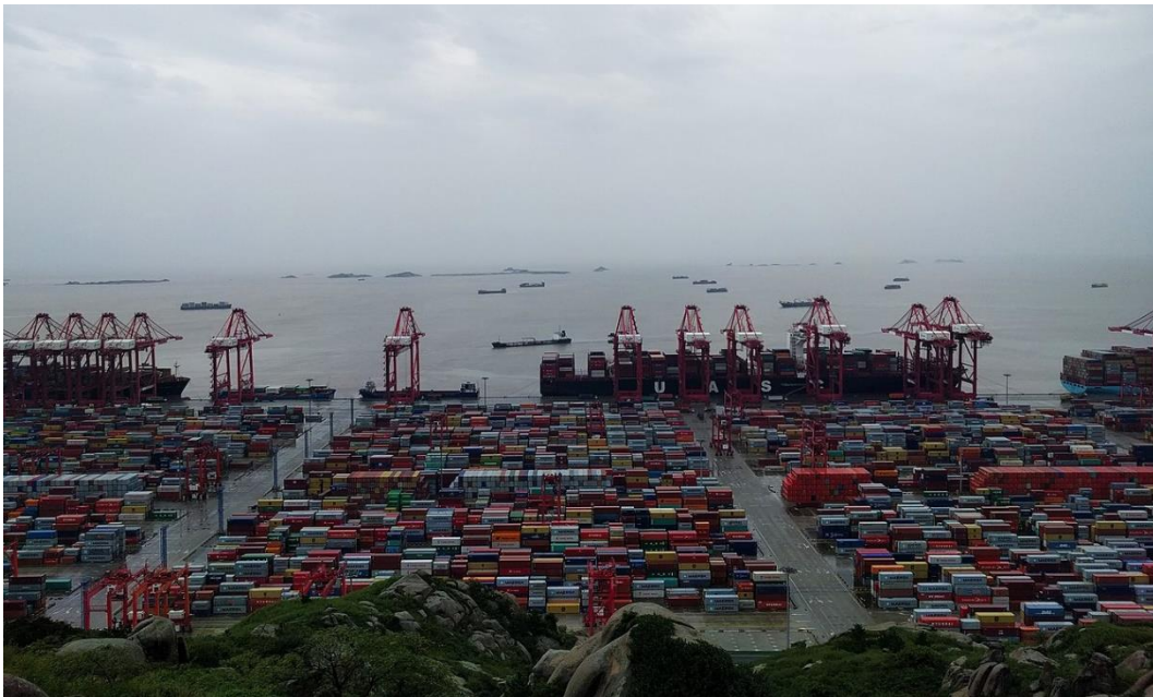
View of the container terminals of the Yangshan Deep Sea Port (photo: Gmbsfd)
